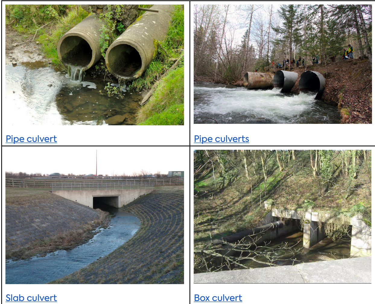
Figure 1: Culvert and Weir Structures
